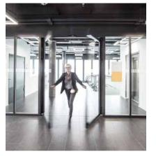
The automatic fire safety sliding doors offer convenient access in day-to-day use and serve as a tested fire barrier in the event of a fire. They can also be fitted with emergency exits to provide a life-saving escape route.
